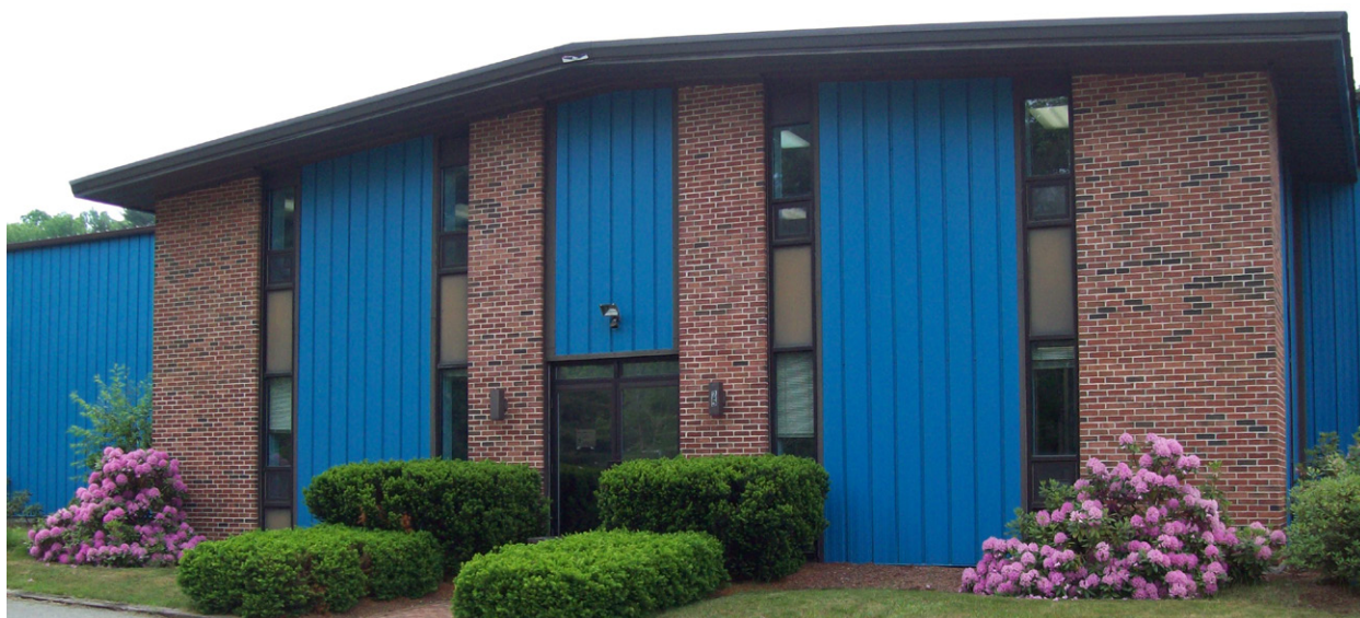
Quality Water Products facility in South Barre, Massachusetts, home of New Concept Tools
